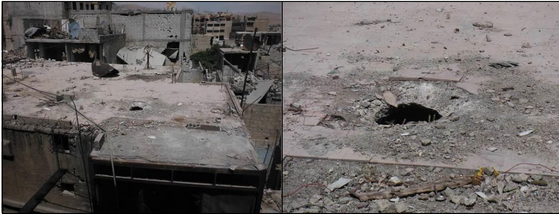
FIGURE A.6.3 ADJACENT ROOF SHOWING A CRATER SIMILAR TO THE ONE ON THE ROOF TERRACE AT LOCATION 2
